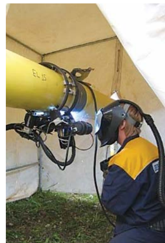
▲ Recent orbital technology monitors several welding parameters simultaneously and records the data for the entire run.
